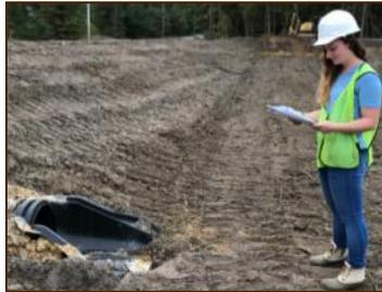
Georgie Grieb checks the placement of a headwall against the construction plans
